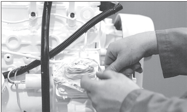
Figure 12: Cover lines, inlets and injection pump outlets.
