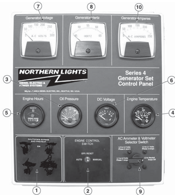
Figure 4: Series 4 B Generator Control Panel
