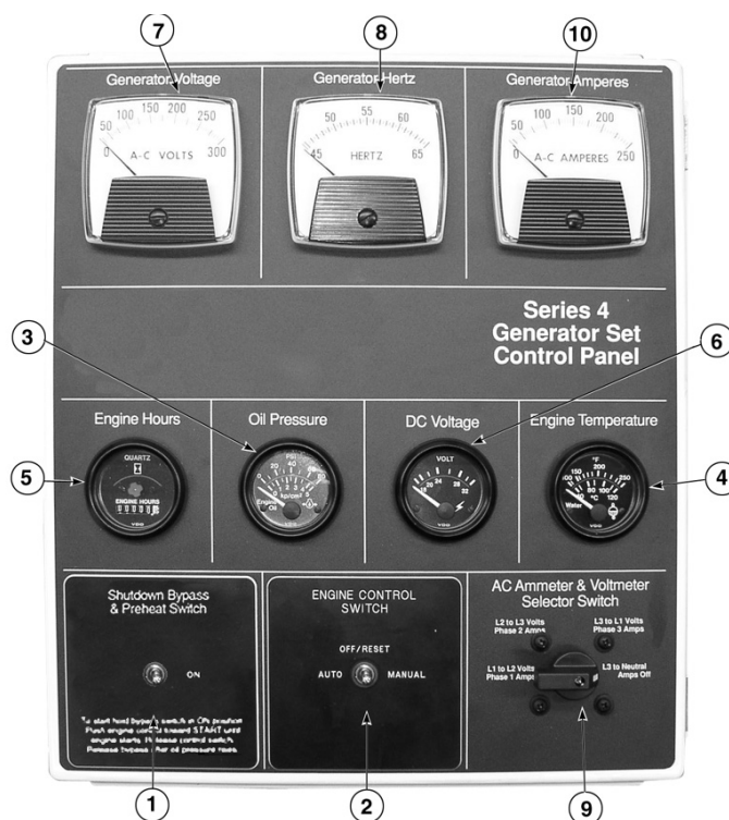
Figure 8: Series 4 B Generator Control Panel
