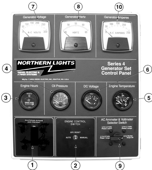
Figure 4-C: Series 4 Generator Control Panel
