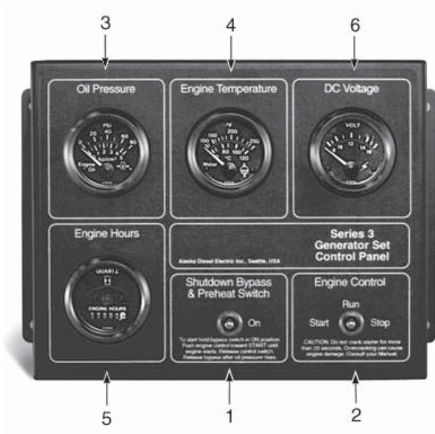
Figure 3: Series 3-B Generator Control Panel
