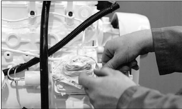
Figure 12: Cover lines, inlets and injection pump outlets.
