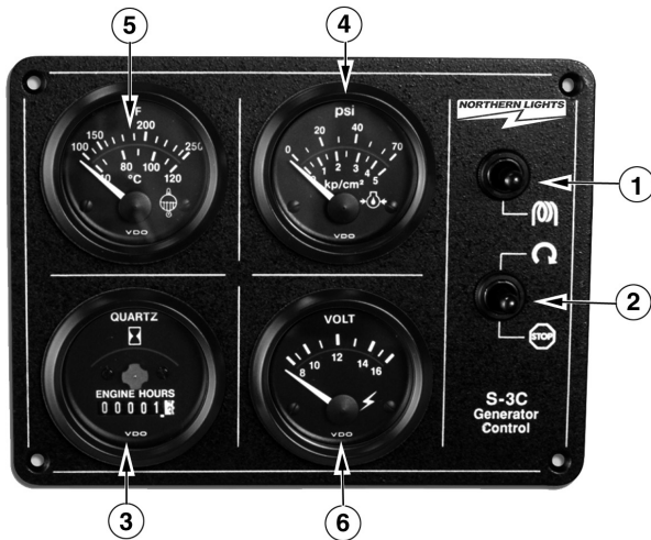
Figure 3-B: Series 3 Generator Control Panel
