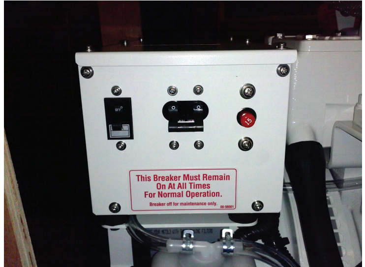
Photo showing completed side panel with regulator breaker, AC output circuit breaker, DC circuit breaker and warning label.
