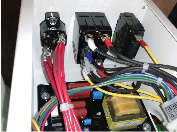
Photo showing connections on DC circuit breaker, AC output circuit breaker and regulator breaker
