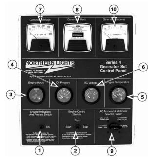
Figure 4-C: Series 4 Generator Control Panel
