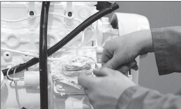
Figure 13: Cover lines, inlets and injection pump outlets.
